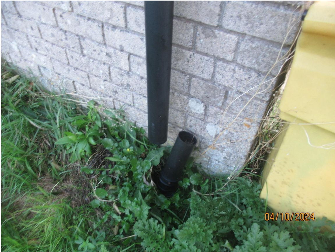
P11 – broken drainpipe
